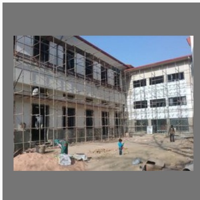
School Building Construction Services
