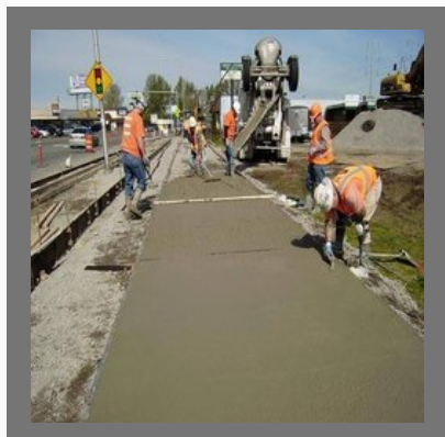
Cement Road Construction Services
