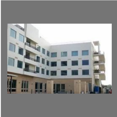
School Building Construction Service
