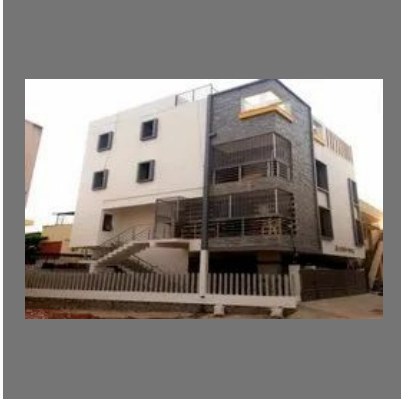
Commercial Building Construction Service
