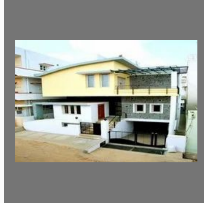
Commercial Projects Construction Service
