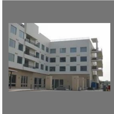
Hotel Construction Service
