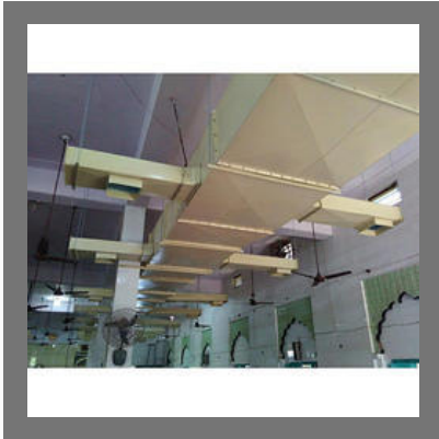
Central Ducting Installation Service
