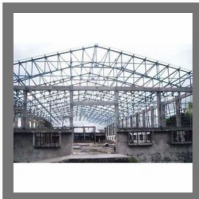
Mild Steel Fabrication Services
