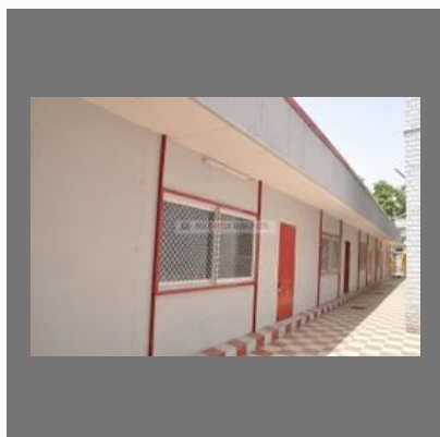
Prefab School Building
