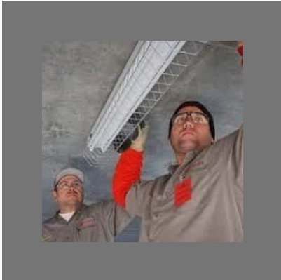
Indoor & Outdoor Lighting Wiring Service
