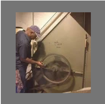
Exhaust Fans Repairing
