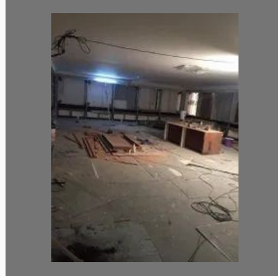
Office Renovation Works
