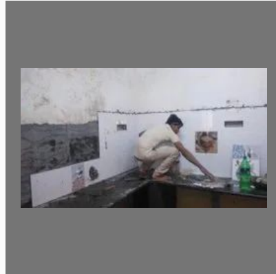
Kitchen Renovation Work
