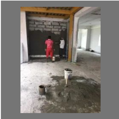
Civil Plastering Work
