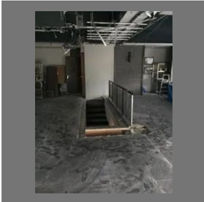
House Renovation Work
