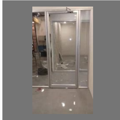
Office Renovation Work
