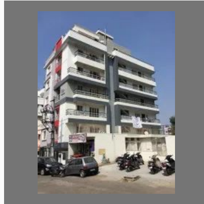
Commercial Painting Works
