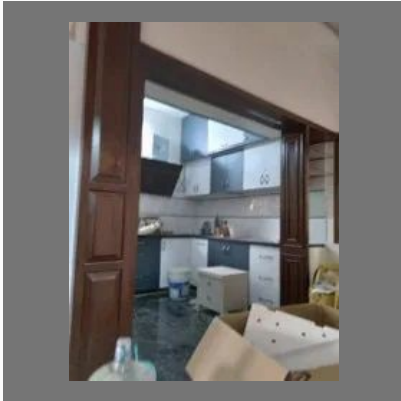
House Interior Work
