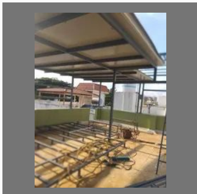
MS Roofing Fabrication Works
