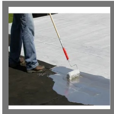
Terrace Water Proofing Services
