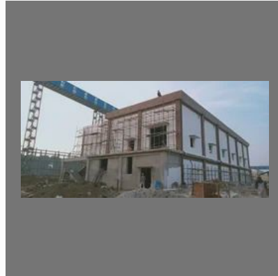
Industrial Wall Painting Service
