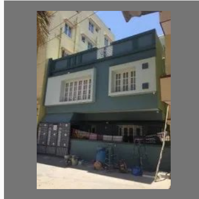
House Construction Works
