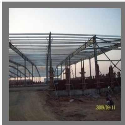
Warehouse Design Services
