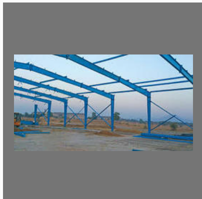
Pre Fabricated Structure
