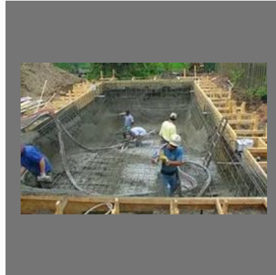
Construct Swimming Pool
