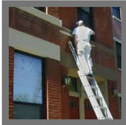
Exterior Wall Painting Services
