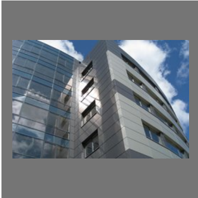
Exterior ACP Sheets
