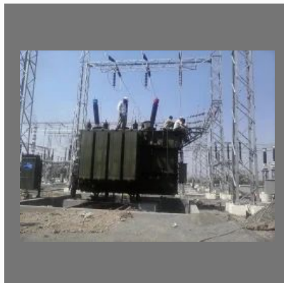
Electrical Erection Service
