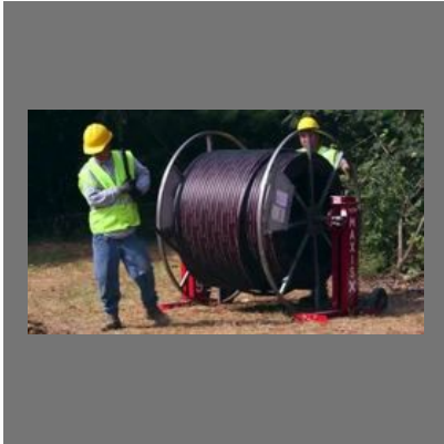
HT Cable Laying Service
