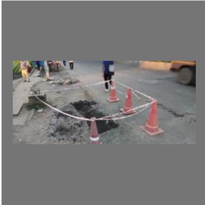
Underground Cable Laying Service
