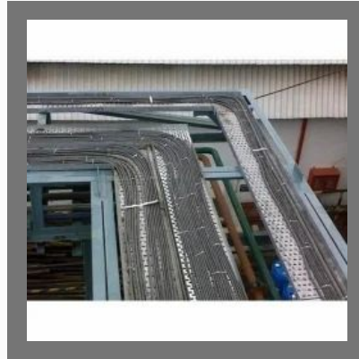
LT Cable Laying Service
