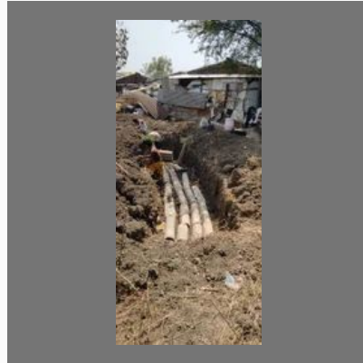
Cable Laying Service
