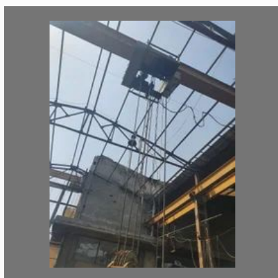
Truss Roofing Shed
