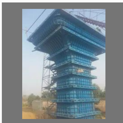
Pier Cap Shutter
