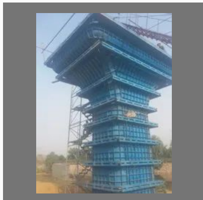
Pier Cap Shuttering
