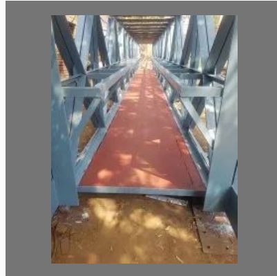
Overhead Bridge Fabrication
