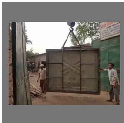
Retaining Wall Shuttering
