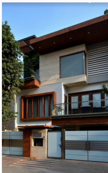
luxury residential villas construction
