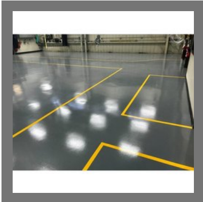
Epoxy Paint Coating Service
