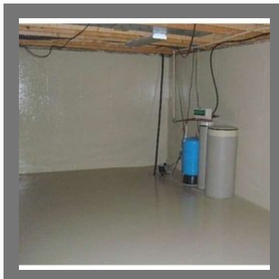
Basement Waterproofing Service
