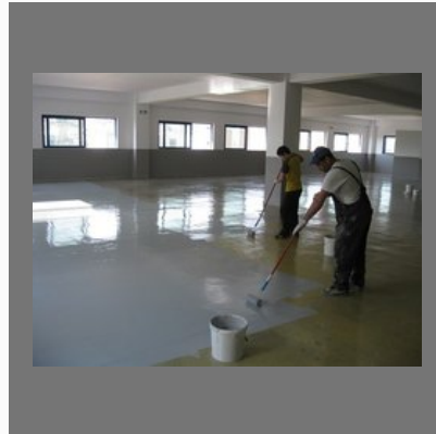
Self Leveling Screed
