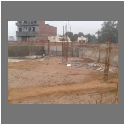
Commercial Construction Service
