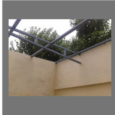
Commercial Construction Service
