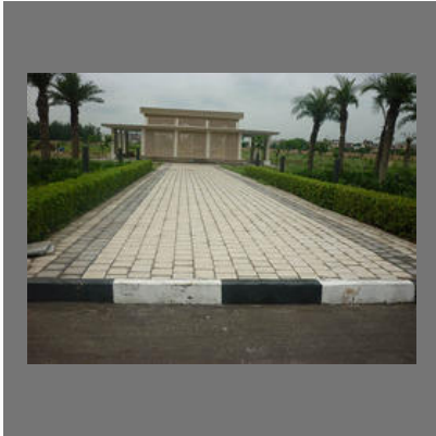
Commercial Construction Service
