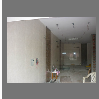
Commercial Construction Service
