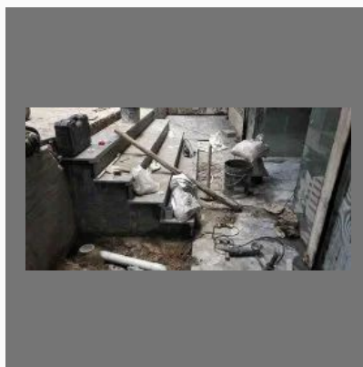
Floor Work - Flooring Services
