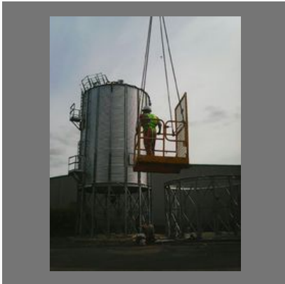
Boiler Erection Service
