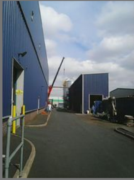
Industrial Prefabricated Shed
