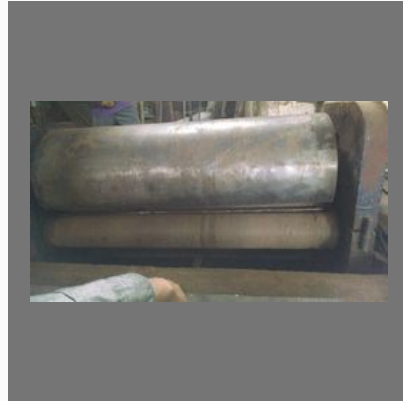
MS Tank Fabrication Work
