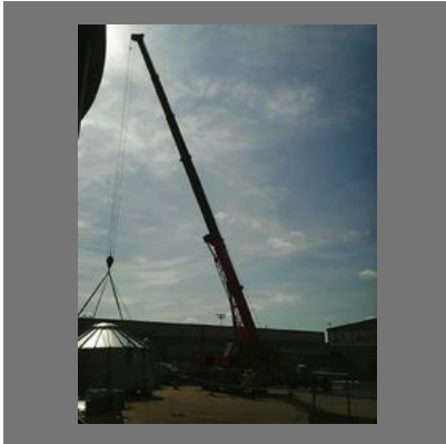
Erection And Commissioning Services
