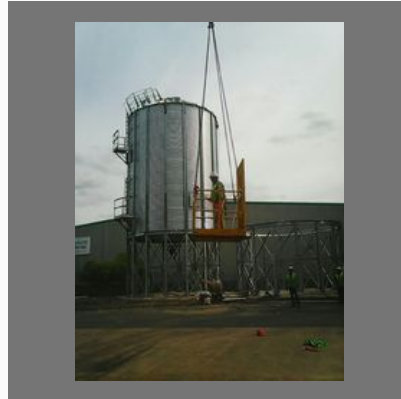
Tank Erection And Commissioning Services
