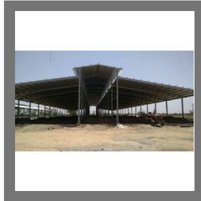
Shade Erection And Commissioning Service
