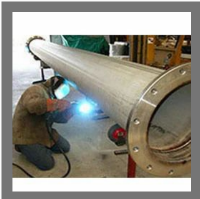
Pipe Line Fabrication Services
