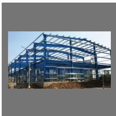
Peb Steel Structure
