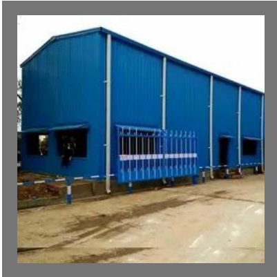
Tin Roofing Shed
