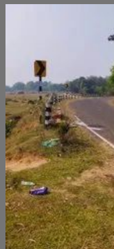
Road Sign Board Installation Service
