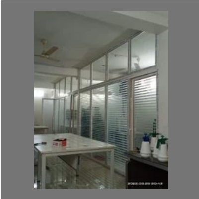
Upvc Office Partition
