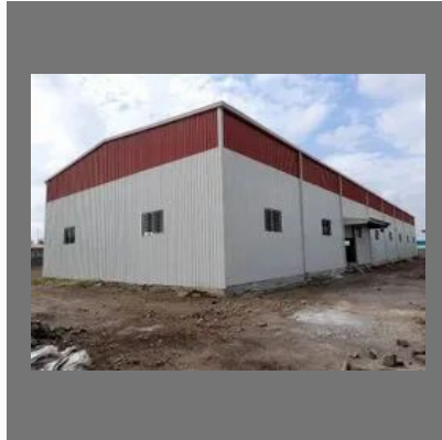
Mild Steel Prefabricated Factory Shed
