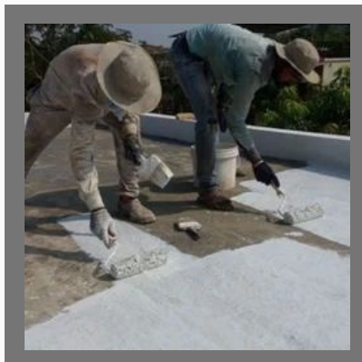
Roof Waterproofing Services In Indore
