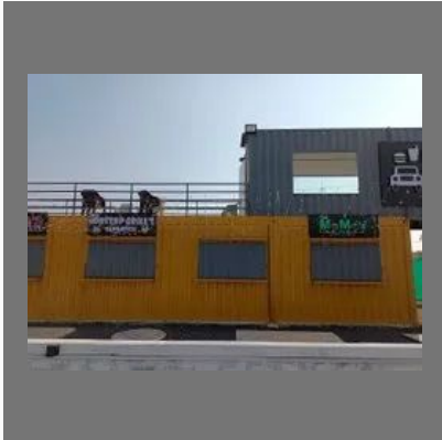
Modular Mild Steel Fabricated Shed
