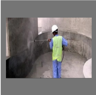
Water Tanks Waterproofing Services
