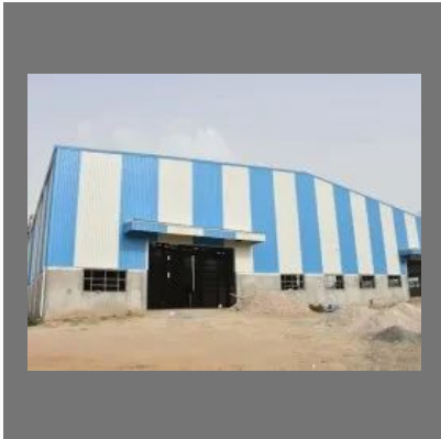
Mild Steel Warehouse Shed
