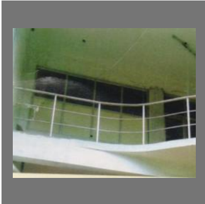
Balcony Hand Rail
