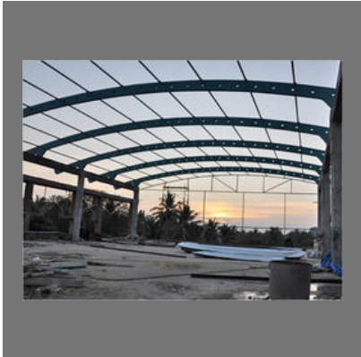
Prefabricated Structure Fabrication Service
