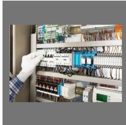
Commercial Building Electrical Work
