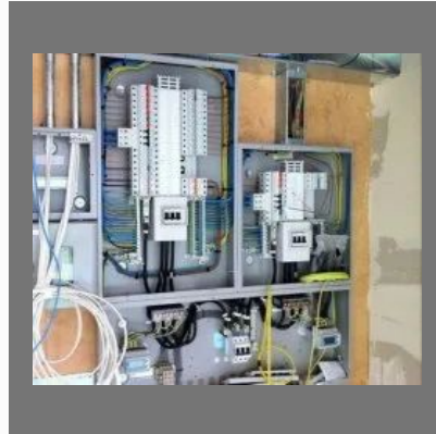
Electrical Wiring Installation Service
