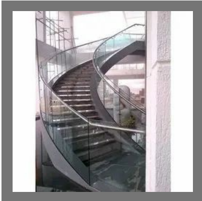
Helical Curved Staircase
