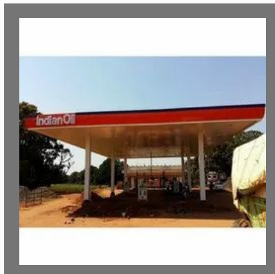
Petrol Pump Canopy
