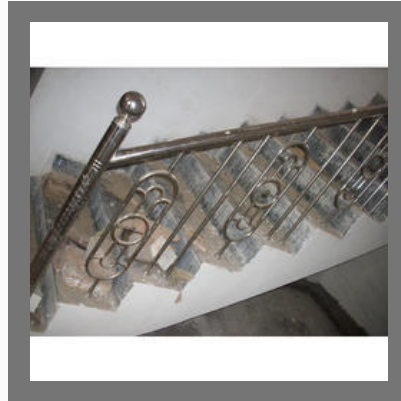
Stainless Steel Pipe Railing
