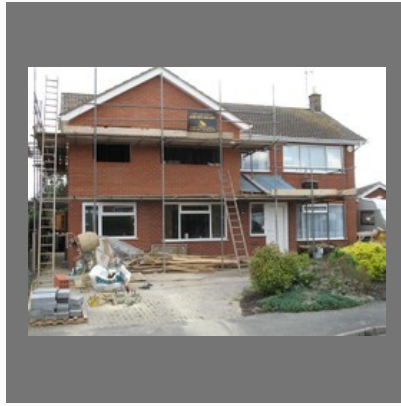
Renovation Work For House
