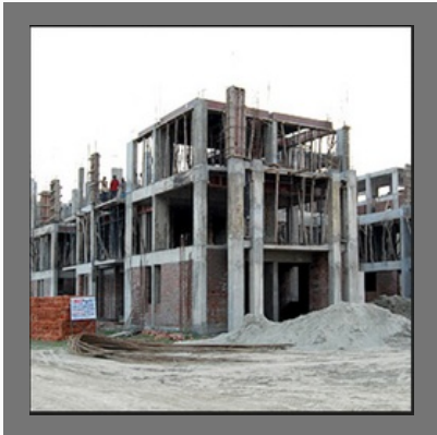
Commercial Building Construction Services
