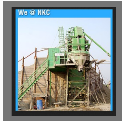
Industrial Building Construction Services
