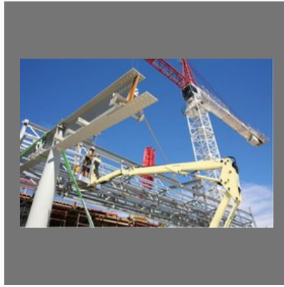
Erection Work Service
