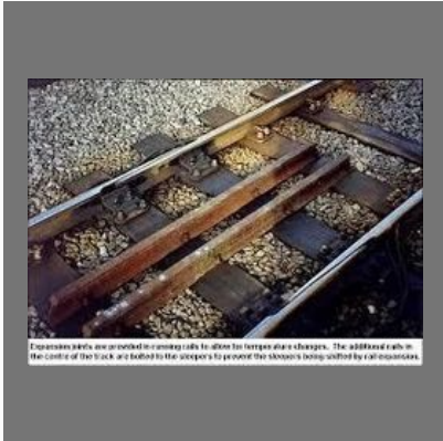
Improved Switches Expansion Joint
