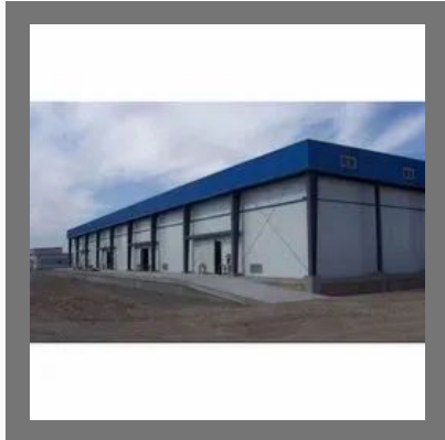
Warehouse Prefabricated Cold Storage Room
