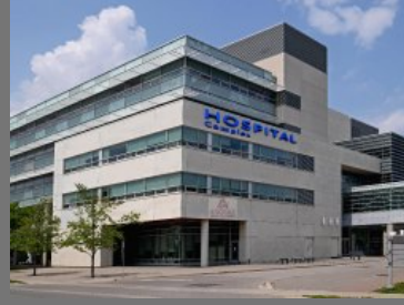
Hospital Building Construction Services
