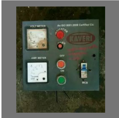
Control Panel Repairing Service
