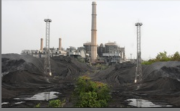
Coal Based Power Stations
