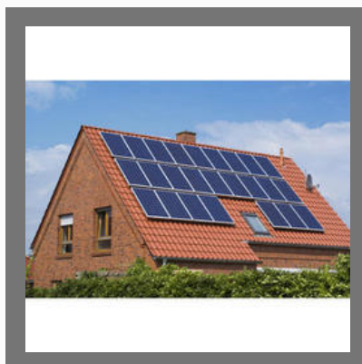
Rooftop Solar Panel
