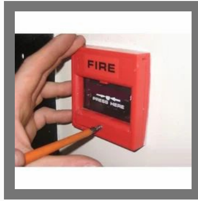
Fire Alarm Installation Services
