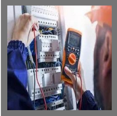
Office Electrical Wiring Services
