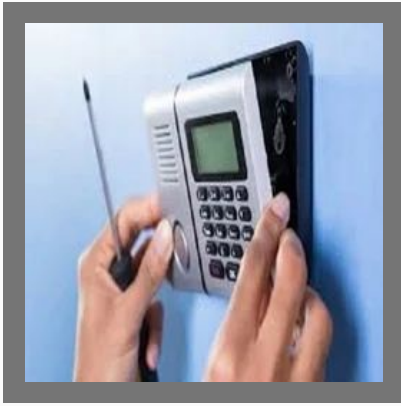
Burglar Alarm System Installation Services
