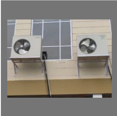
Air Conditioner Installation Services
