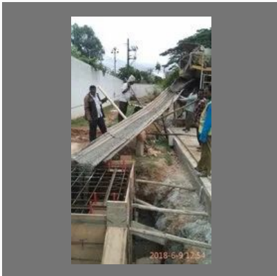
Residential building construction
