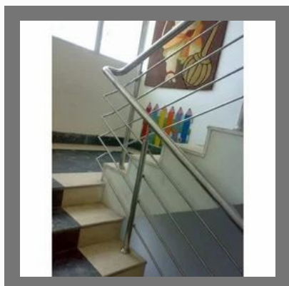
Stainless Steel Stair Railing
