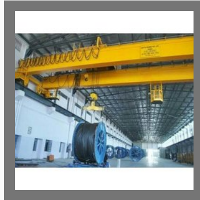
Double Girder Eot Crane
