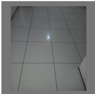
Floor Tiles Fitting Services
