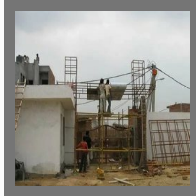
House Construction Services
