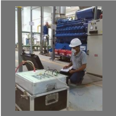
HT Motors Electrical Testings
