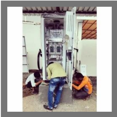
EV Charging Station Installation Service
