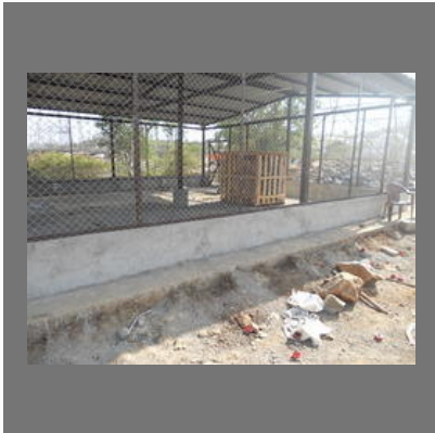
Civil Work Services
