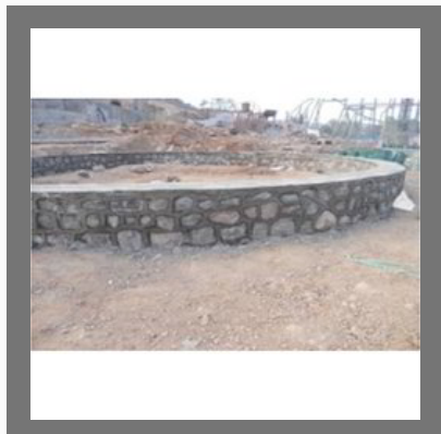
Industrial Construction Services
