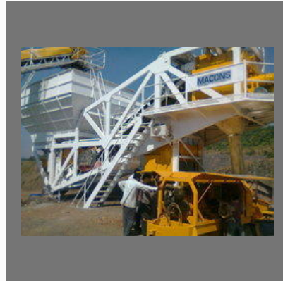
RMC Plant Set Up on lease
