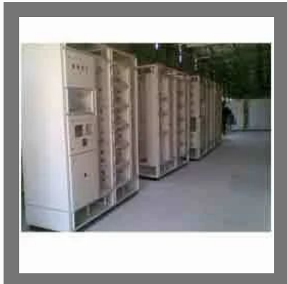
Enclosure Panel Fabrication
