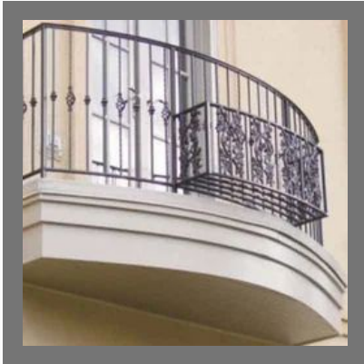
SS Grill Fabrication
