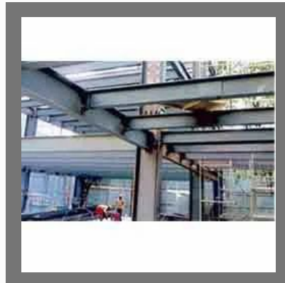
MS Heavy Truss Work
