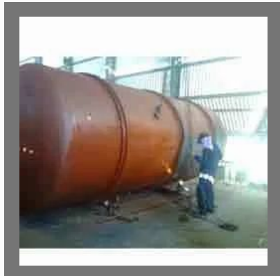
MS Storage Tank Fabrication
