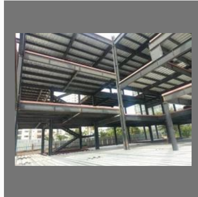
Roof Decking Sheets
