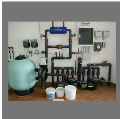
Sewage Treatment Plants
