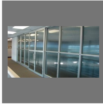
Aluminium Partition Works
